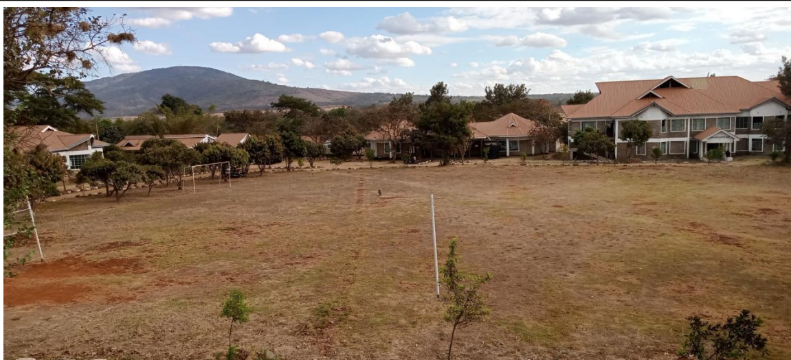
An aerial view of CSAEA with Kilimambogo hills in the background. Much of the work on new office, sports and accommodation infrastructure was concluded in the period in review.
